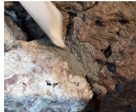
FIGURE 2 APPLYING SAND/CEMENT MIX
